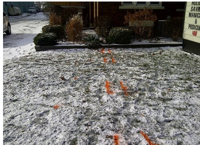
Fig. 1— Locates marked before drilling
