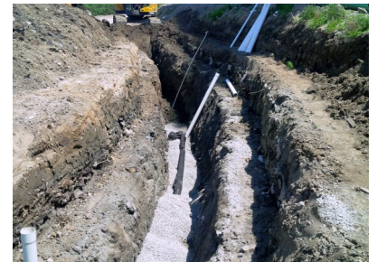
Fig. 2—Installation of passive venting system
